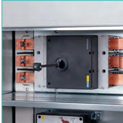
Separation of functional compartments according to user requirements
