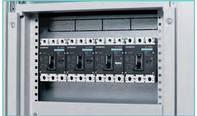
Outgoing feeders set with SENTRON 3VL circuit breakers
