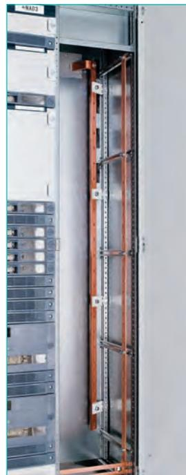
The vertical PE and N busbars are located on the right side of the cable compartment.
